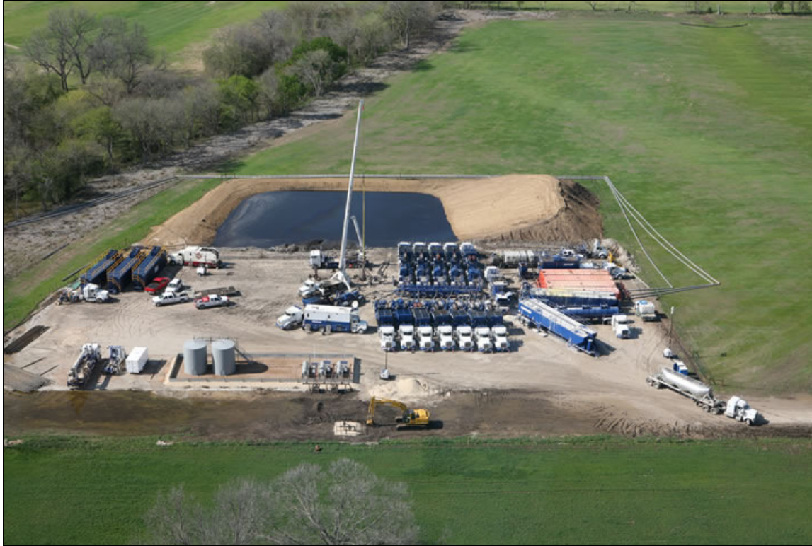
Figure 2 - Barnett Shale frac job in progress 7 .
